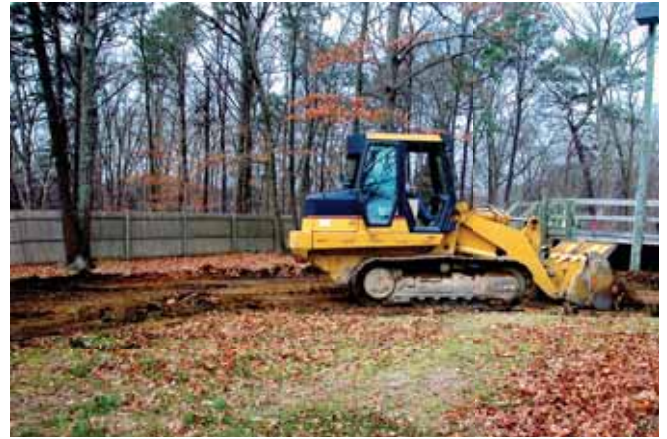
Figure 27-4. Grading may be necessary to level the ground in some settings.
