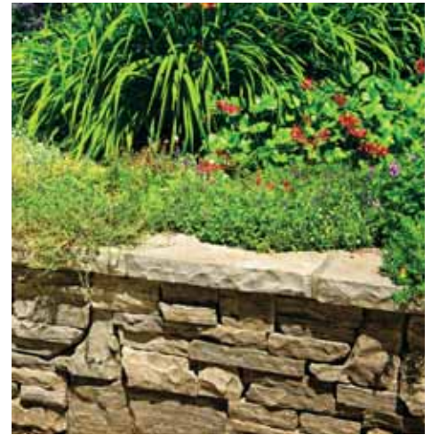
Figure 27-9. Caps finish off a wall in an elegant and functional way.
